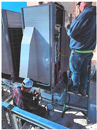
Hook up and Start up of roof units for mechanical systems, the HVAC is currently in programming stage but has been operational for 2 months.
