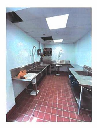
Finished dishwasher area, plumbed and electrical elements connected
