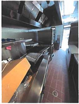
Cook line set, gas regulators and all plumbing electrical installed. Currently proceeding with the hood start up including ansul system, test and balance, and all fire related tasks needed for final inspections.
